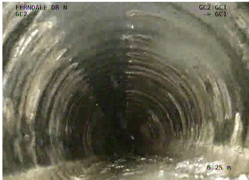
Photo 17: Typical conditions within Gallery approximately 12m downgradient of GC2 showing clogged perforations
