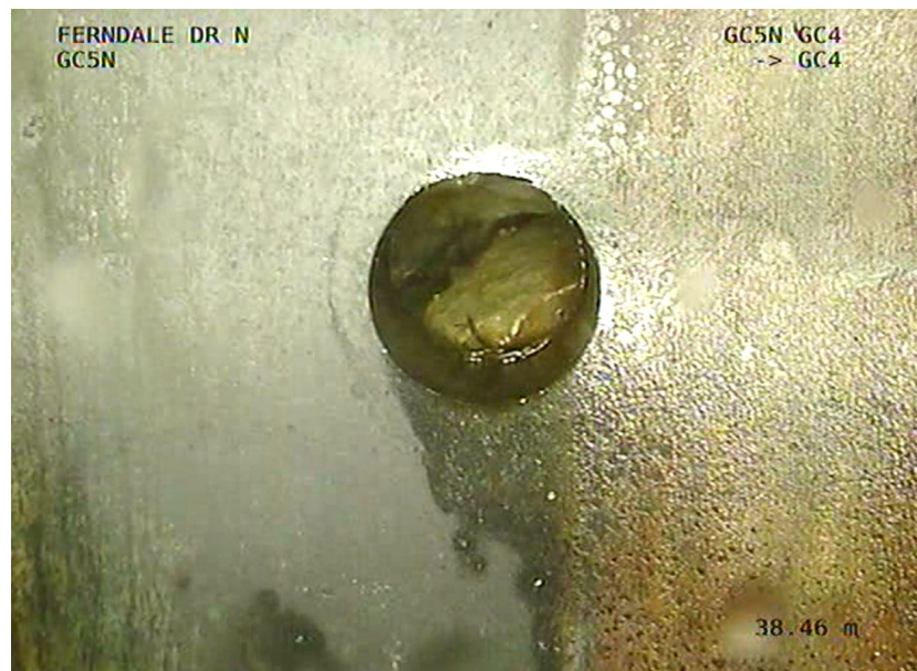
Photo 15: Perforations in the sidewall of the Gallery collector pipe between GC5N and GC4.
