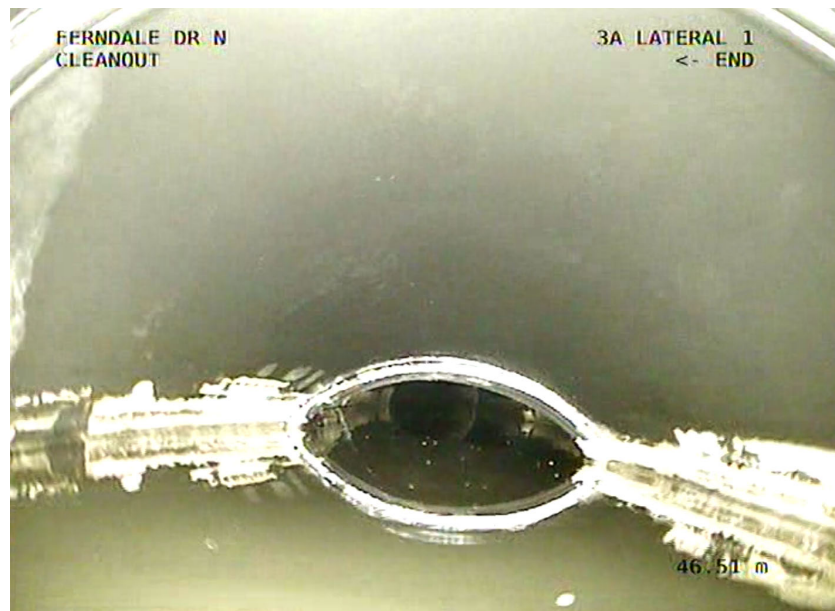
Photo 2: Sumping (as observed in 2020) within west cleanout access to 3A Lateral 1 at approximately 47 m.
