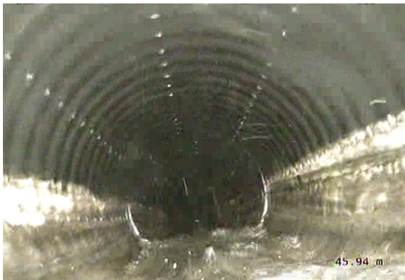
Photo 18: Typical conditions within Gallery between manholes GC2 and GC1 following flushing.
