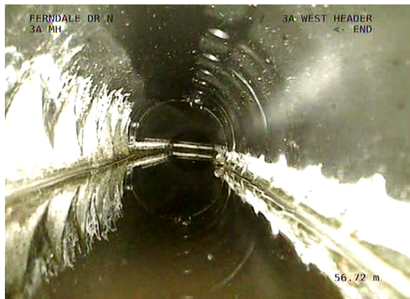
Photo 3: Sumping (as observed in 2020) within 3A West Header at approximately 57 m.
