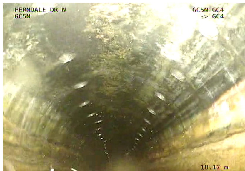
Photo 14: Typical conditions within Gallery between manholes GC5N and GC4 following flushing.
