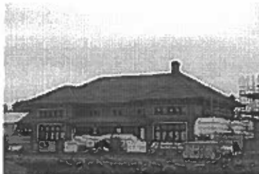
285 Bradford Street "Allandale Train Station" By-Law 2009-144 Aug10/09
