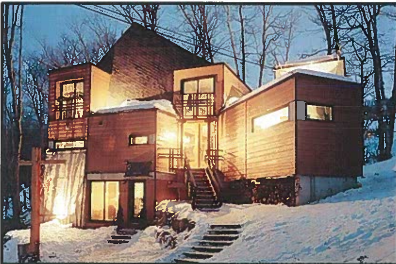
5. Container House – Quebec, Canada
