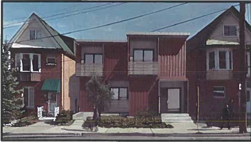
4. Container House (Under Construction) – Hamilton, Ontario
