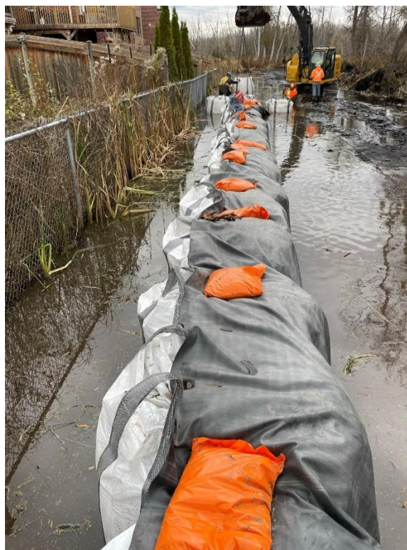
2 October 2023 - Construction of cofferdam
