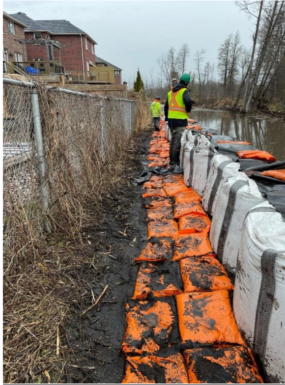
3 November 2023 -Coffer dam after completion and first pump out
