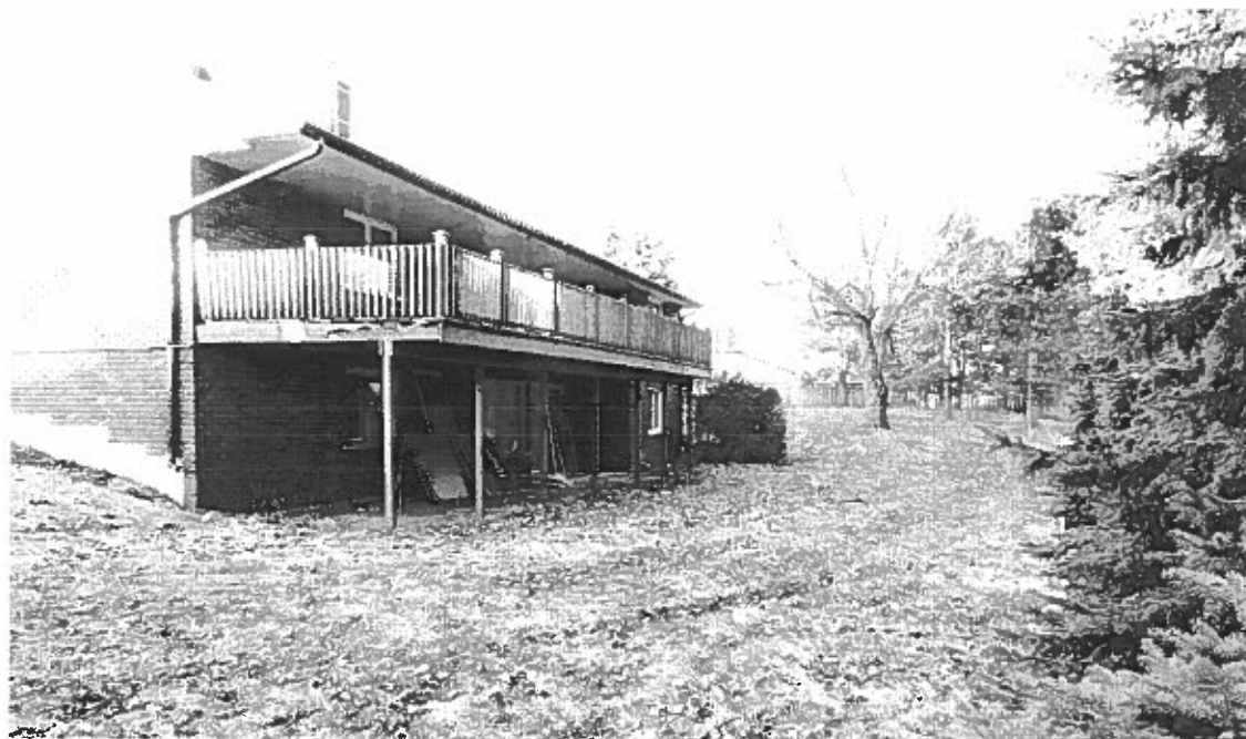
Photograph 1: Walk-out basement, 401 Essa Road, Barrie, ON, looking south
