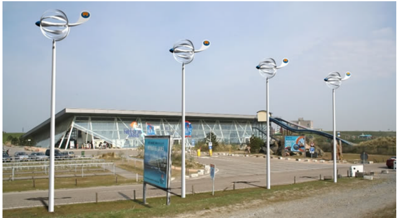
Example of a wind turbine and solar energy installation for street lighting
