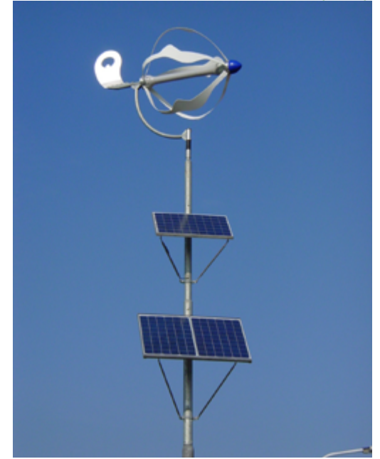
Example of a wind turbine and solar energy installation for street lighting
