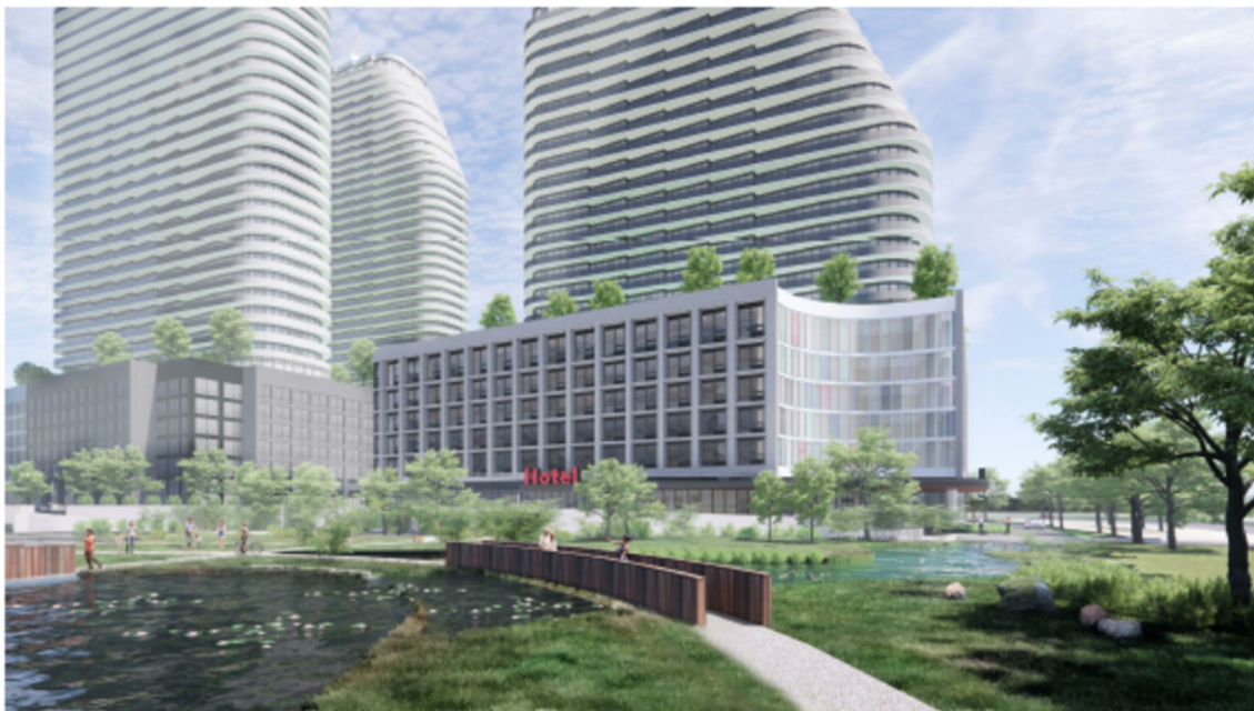
VIEW FROM OPEN SPACE LOOKING NORTH
