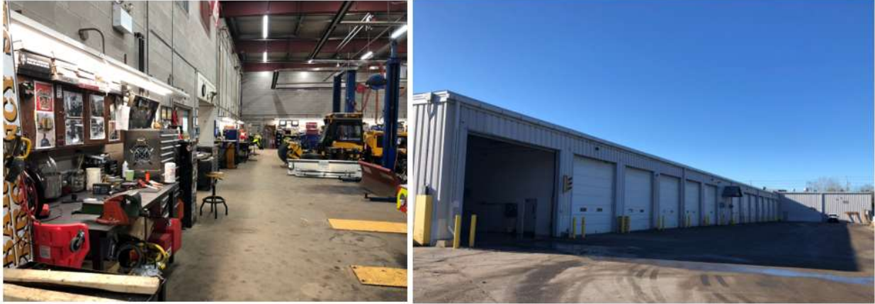
Figure 5 Maintenance Shop Inside (Left) and Outside Rear (Right)
