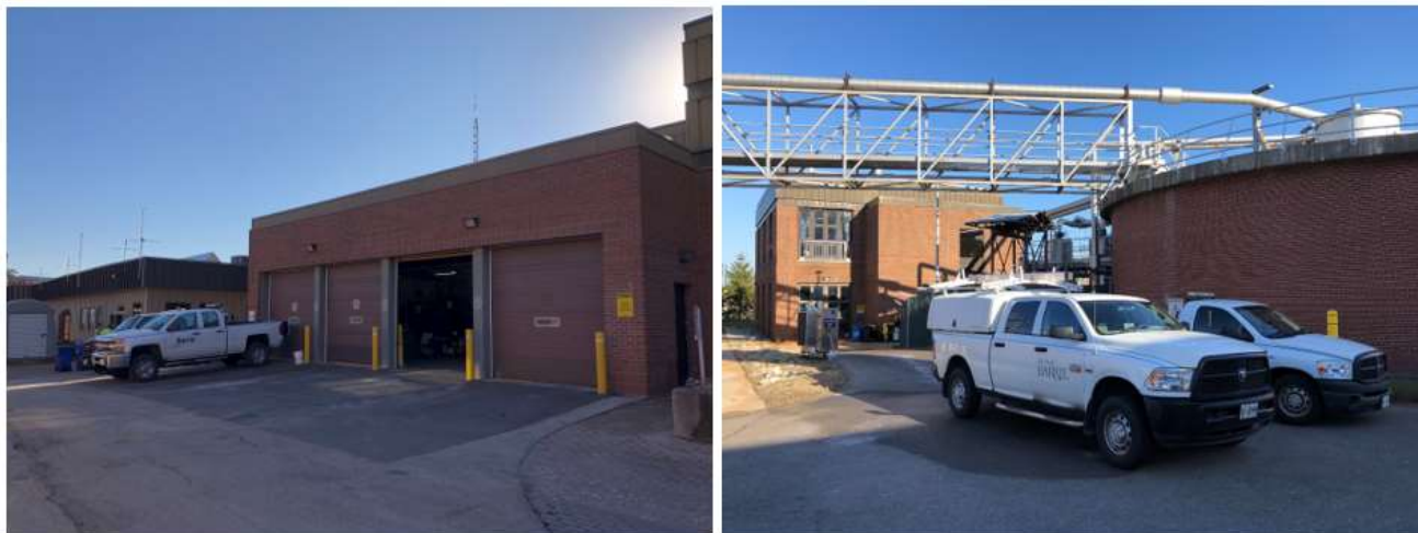
Figure 8 Wastewater Treatment Facility (249 Bradford Street)
