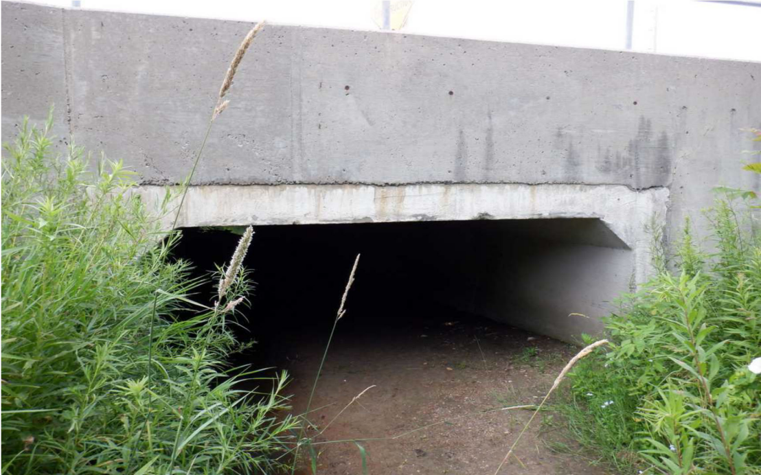
Figure 25 - Typical Bridge Condition Photo
