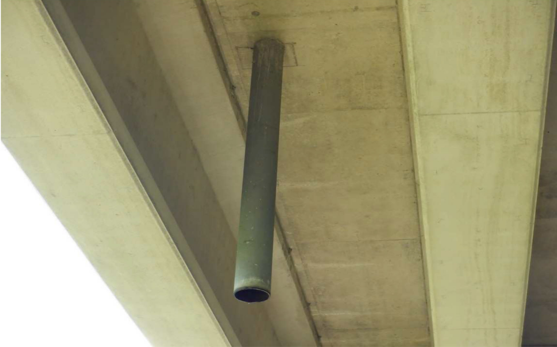
Figure 24 - Typical Bridge Condition Photo
