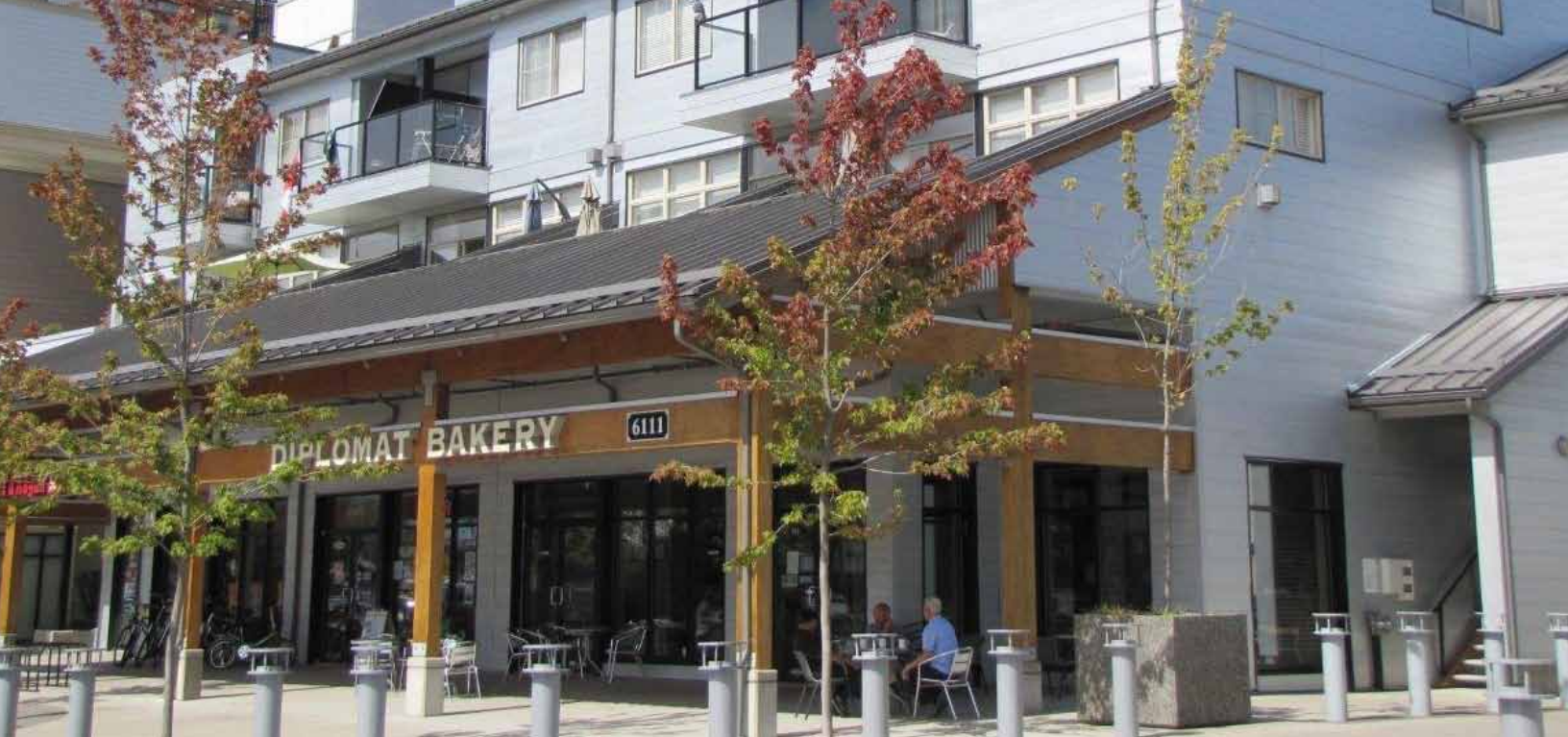
Mixed use buildings should be designed to animate the street frontage and create interaction between indoor and outdoor spaces.
