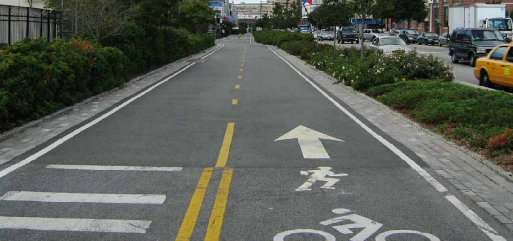
Pathways should be at least 3.0 metres wide, with pedestrian amenities such as lighting, seating and waste receptacles.
