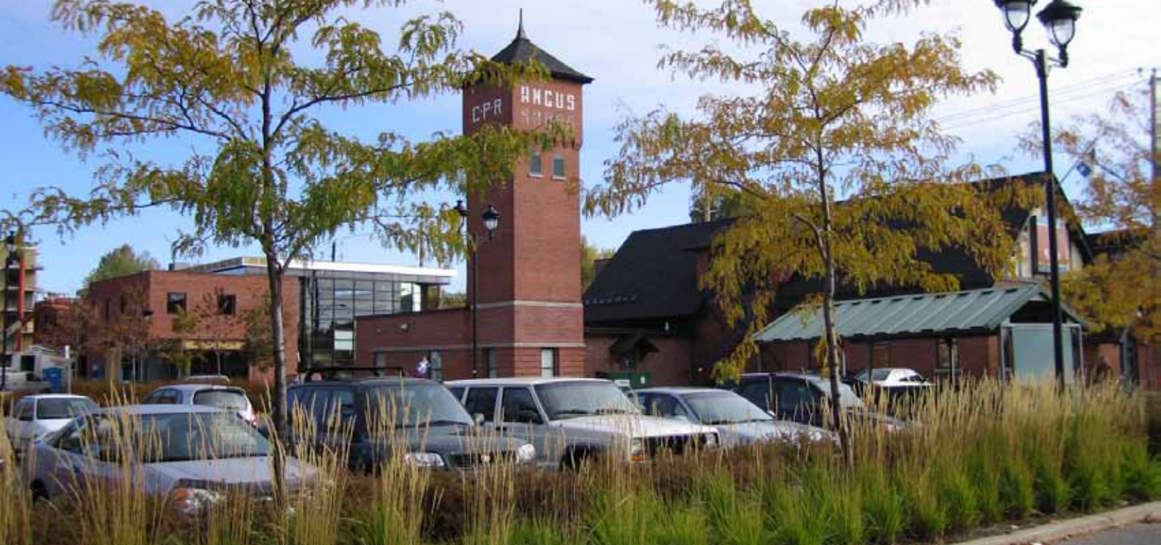
Screening may include low fences, walls and/or landscaping, and should be designed to reflect safe community design practices.
