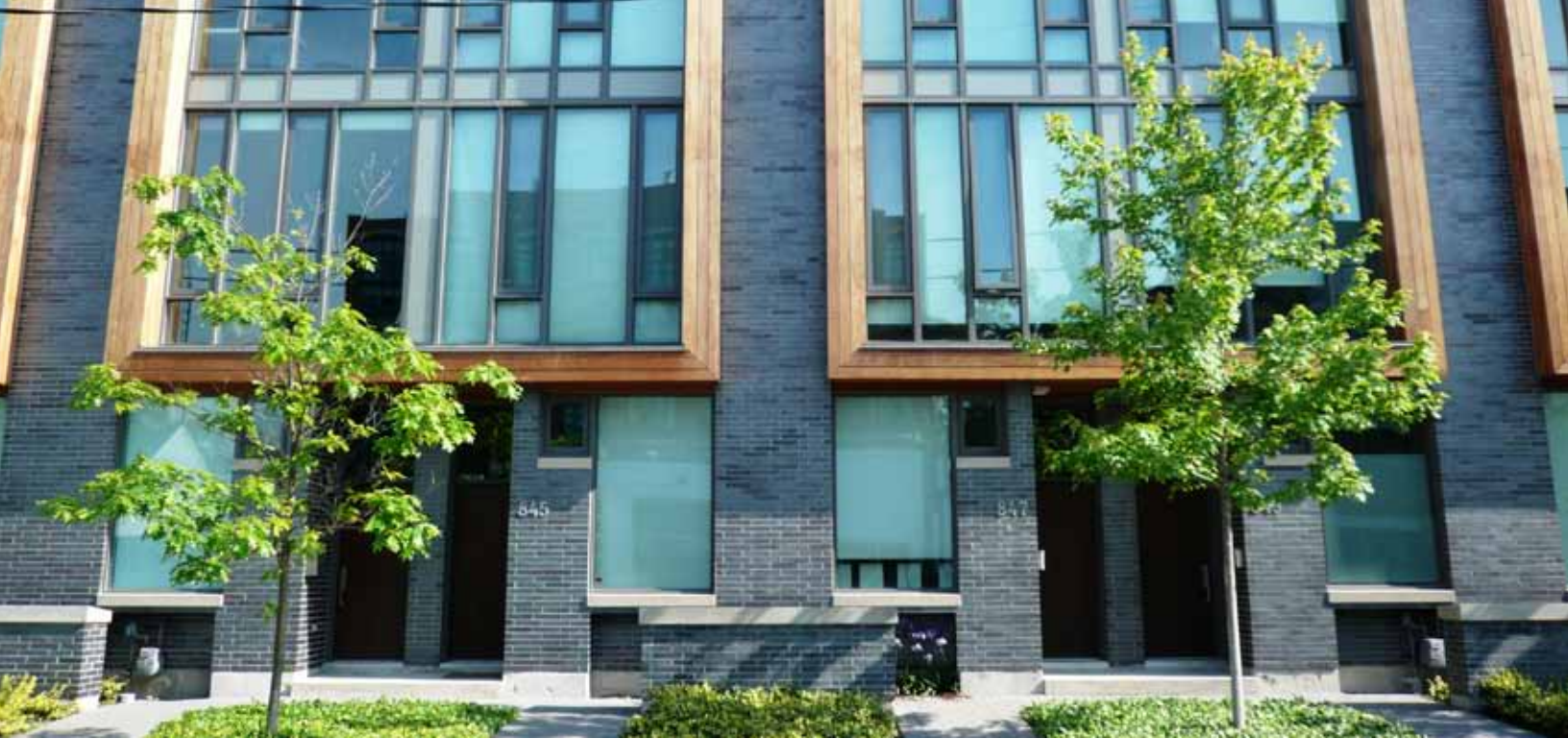
Buildings should establish a specific and unique character and conform to heights and densities identified in the Secondary Plans.
