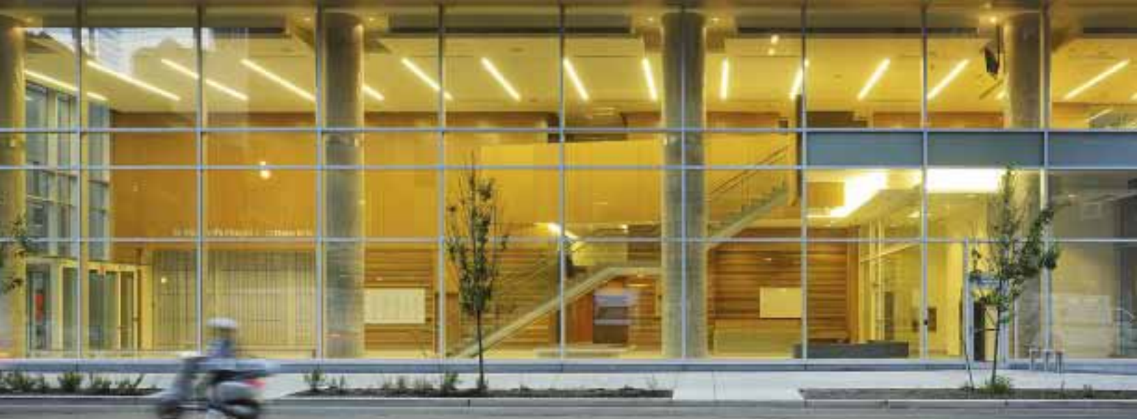
Glazing and well-lit building entrances promote visibility and surveillance to promote safety.
