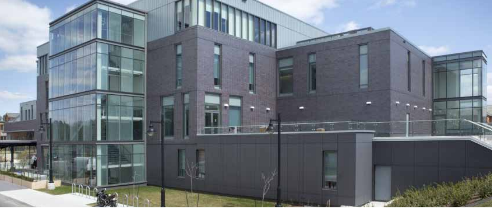
Office buildings with long facades should be articulated with multiple unit entrances and architectural details.
