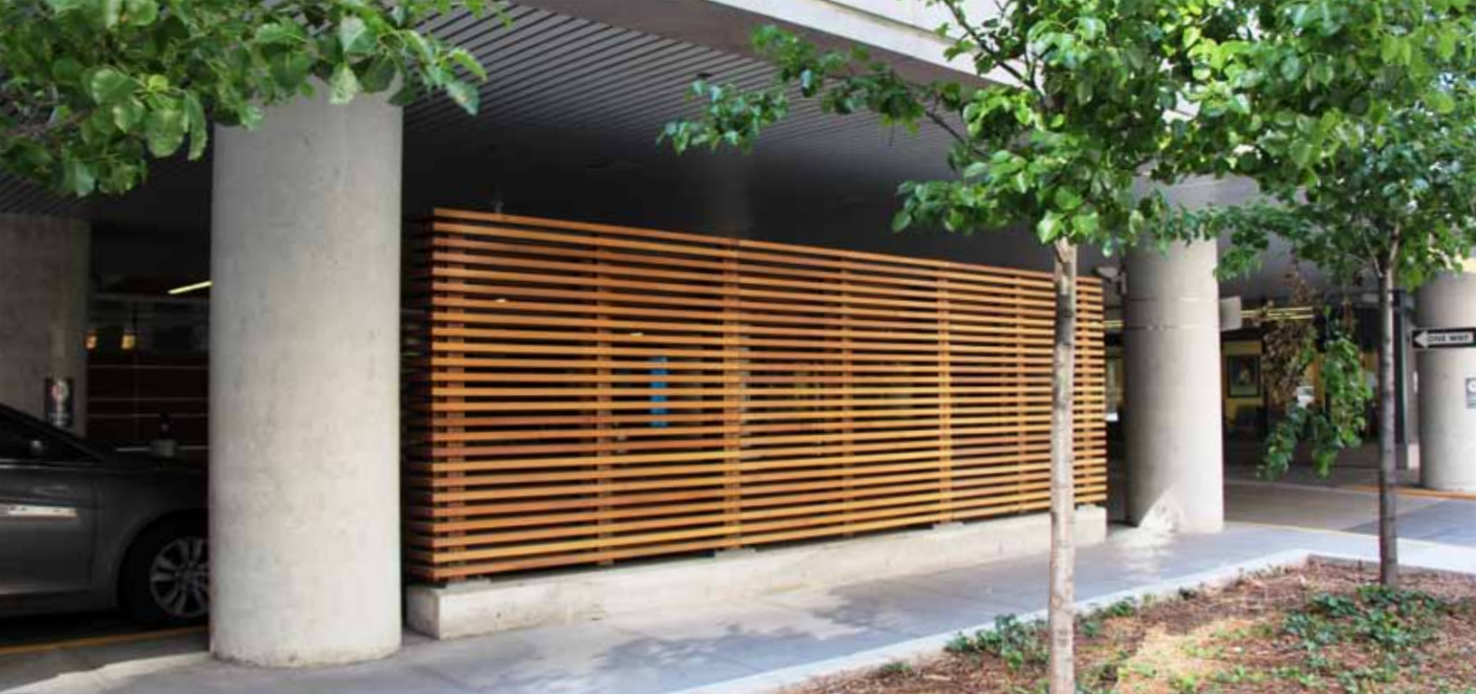
Servicing and loading areas should be located to the rear of buildings, and screened with high quality, complementary materials.
