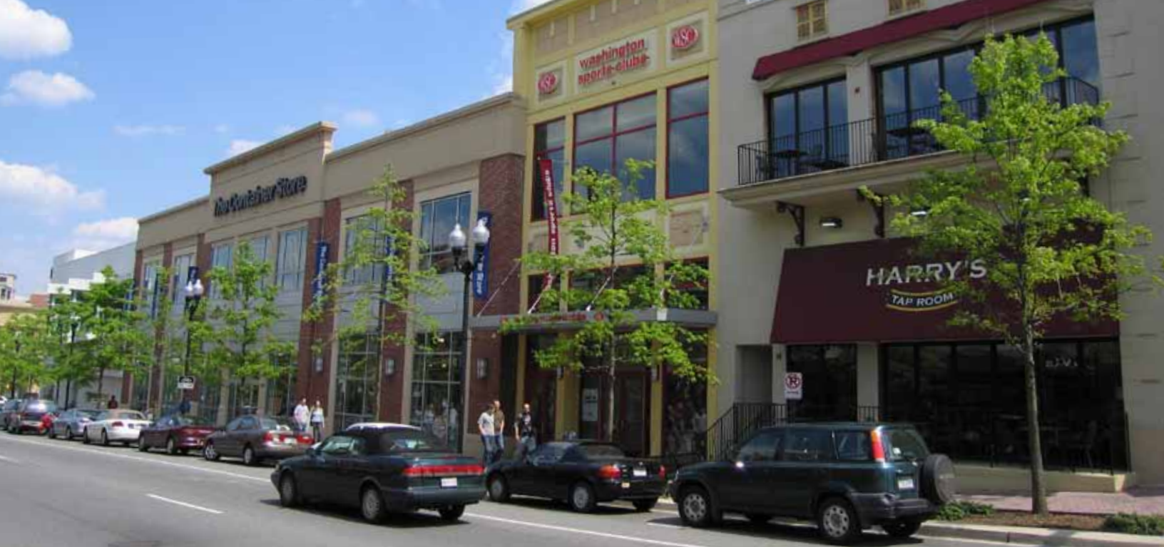
Streetscape design should respond to adjacent land uses, providing enhanced pedestrian space and amenities in high volume pedestrian areas.
