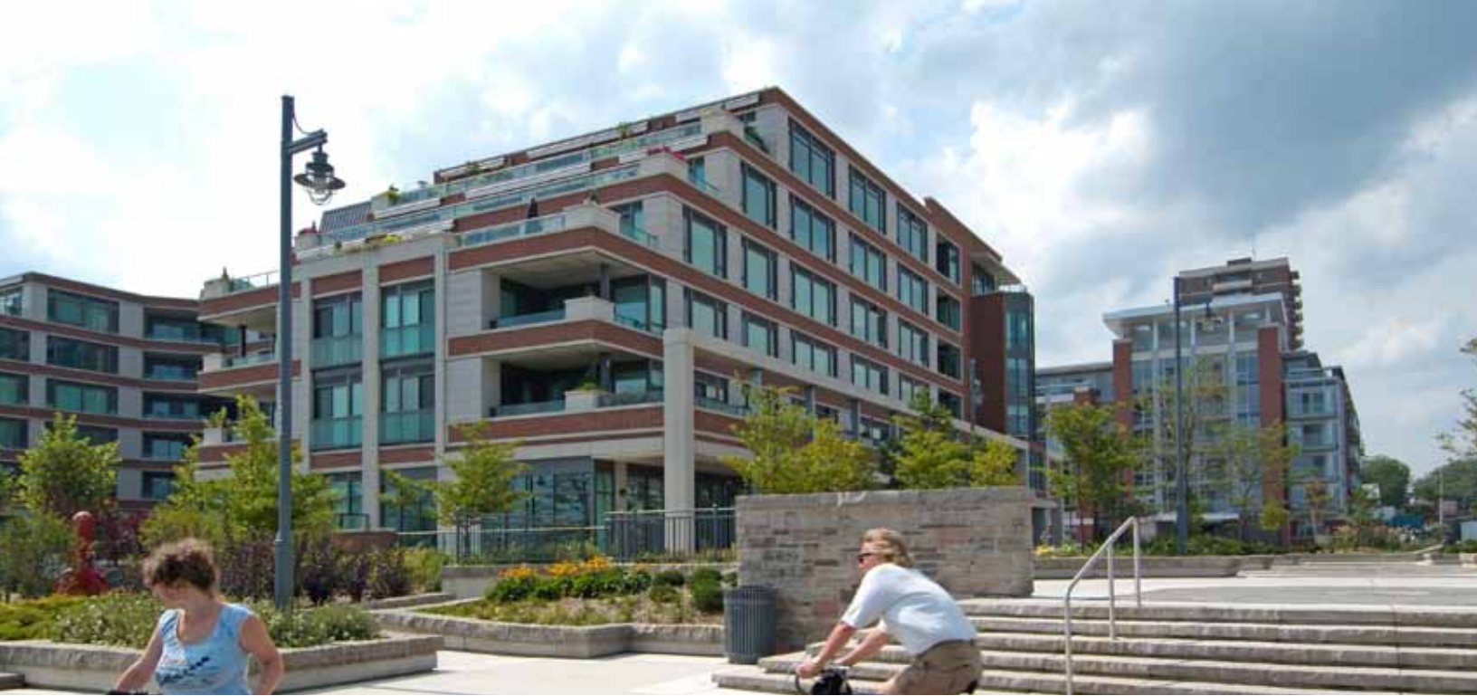
Apartment buildings should incorporate horizontal and vertical articulation elements.
