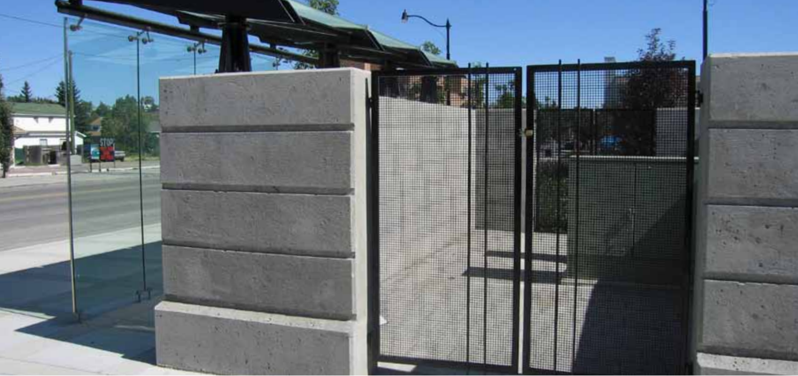
Utility locations should be screened from view when integration into the building design is not feasible.
