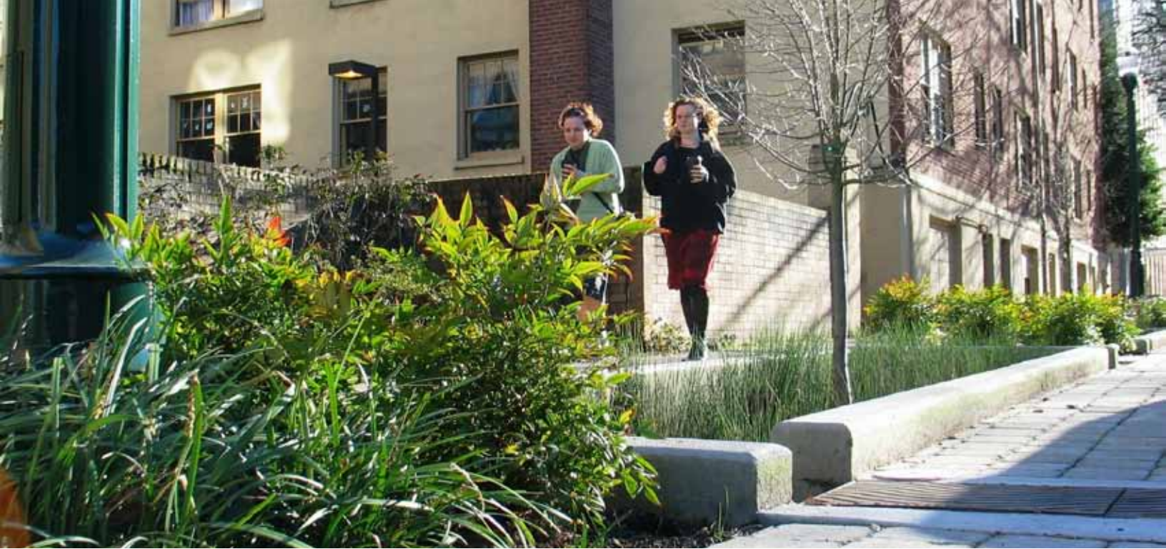
Low impact development measures can be integrated into street design as part of the stormwater management system
