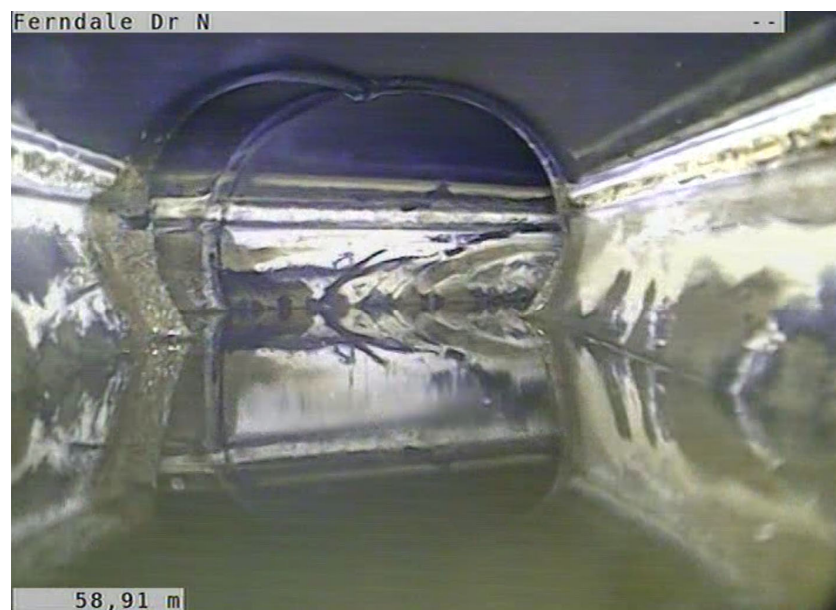
Photo 3: Sumping (as observed in 2019) within 3A West Header at approximately 59 m.
