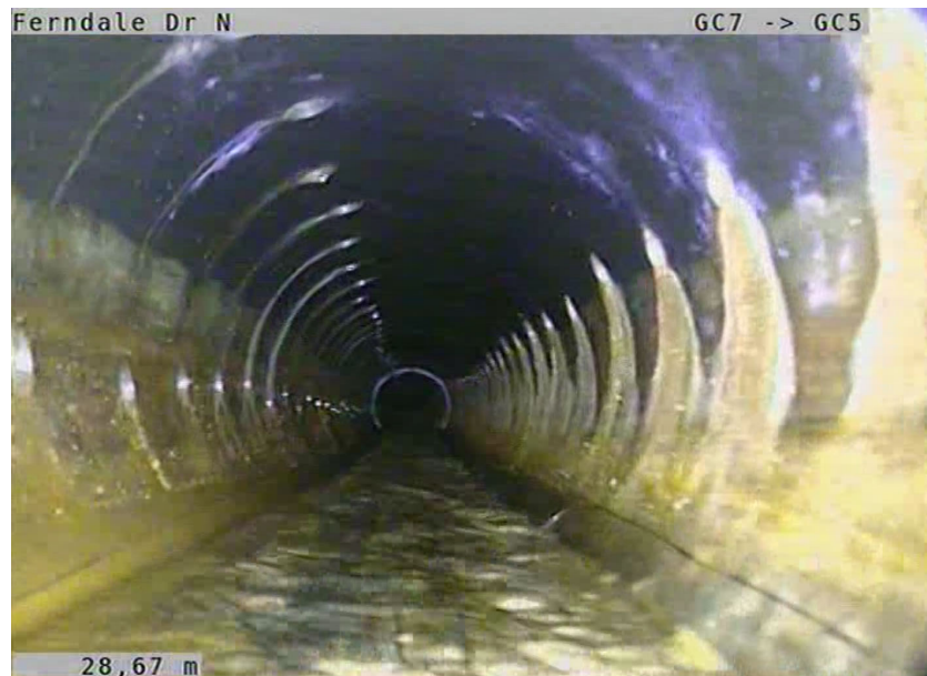
Photo 12: Typical conditions within Gallery between manholes GC7N and GC5N following flushing.
