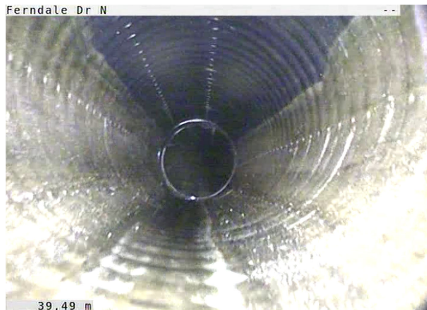
Photo 17: Typical conditions within Gallery between manholes TDMH1 and GC2 following flushing.
