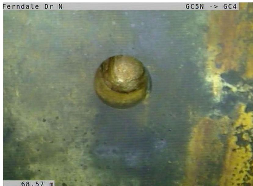
Photo 13: Perforations in the sidewall of the Gallery collector pipe between GC5N and GC4.
