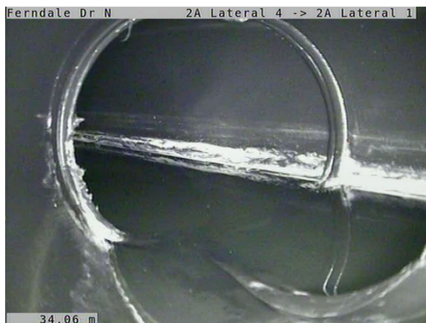
Photo 1: Typical cleanout connection to LCS laterals in Cells 2A and 3A.
