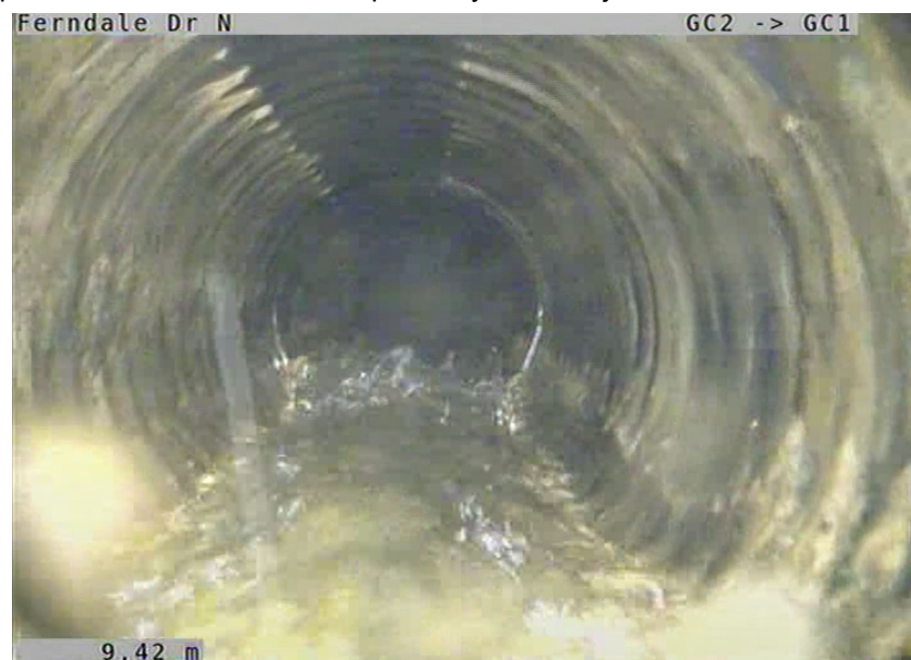
Photo 15: Typical conditions within Gallery approximately 12m downgradient of GC2 showing clogged perforations
