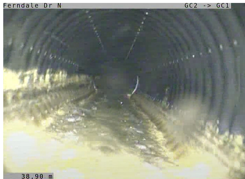
Photo 16: Typical conditions within Gallery between manholes TDMH1 and GC2 following flushing.
